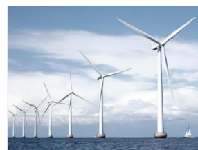
Wind Storage(220V, 10KW)
