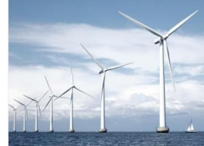
Wind Storage(220V, 10KW)
